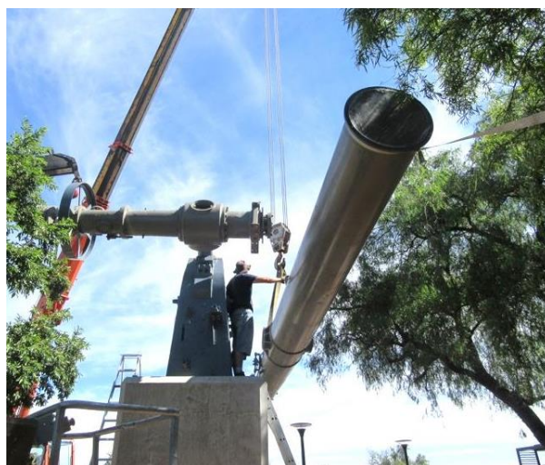
Reassembly of the 27-inch Lamont refractor.
