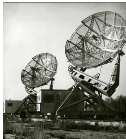
Figure 3: The two equatorially-mounted Würzburg antennas at Nançay were movable on rail-tracks (Image courtesy Paris Observatory).
