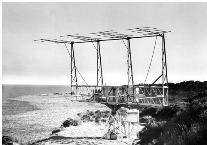
The 'sea-cliff' interferometer at Dover Heights, located north of Sydney's Bondi Beach. At sunrise, on 26 January 1946, Ruby Payne-Scott conducted the first known radio interferometric observation using this device. (Image courtesy National Radio Astronomy Observatory)
