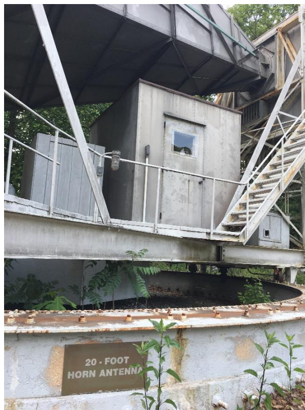
Close-up view of Holmdel Horn showing identifying sign, stairs, and equipment cab, c. 2023. (Image courtesy Jonathan Schilling (CC-SA 4.0), via Wikimedia Commons https://commons.wikimedia.org/wiki/File:Holmdel_Horn_Antenna_close-up_with_20-foot_sign.jpg )
